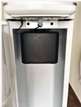
Fig. 5: Interior of the AQA drink Pro 20 cabinet with wastewater tank in place
